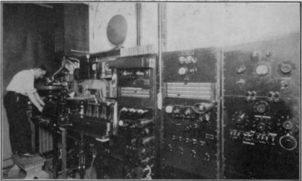
A view of the control panels of the electrical recording system used in studio recording. At the left an operator is seen observing the master wax disc upon which sound vibrations are recorded with means readily available for controlling the amplifying apparatus of the record cutting mechanism.
